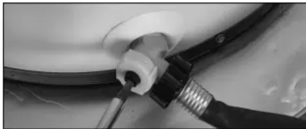
Figure 42 - Draining the water heater.
