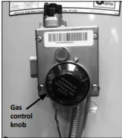
Figure 17 - Turn gas control/temperature knob OFF.
