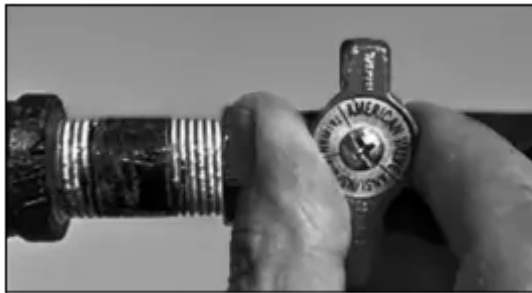
Figure 50 - Gas valve in "off" position.
