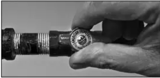
Figure 32 - Gas valve in "on" position
