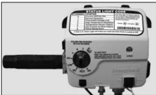
Figure 56 - Gas control/valve with threaded pipe.
