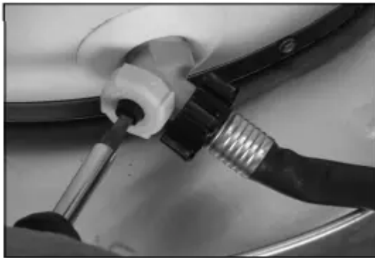
Figure 20 - Draining the old water heater.
