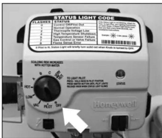
Figure 40 - Turn gas control/temperature knob OFF.
