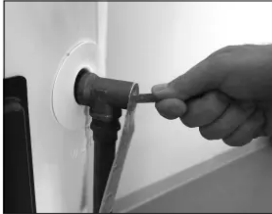
Figure 38 -T&P Relief Valve
