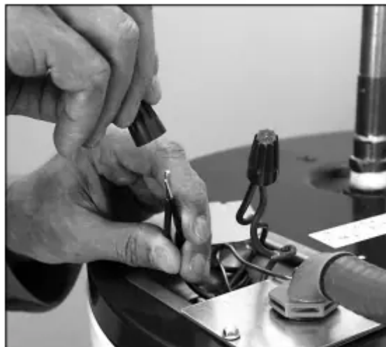
Figure 19 - Connecting the electrical wires.
