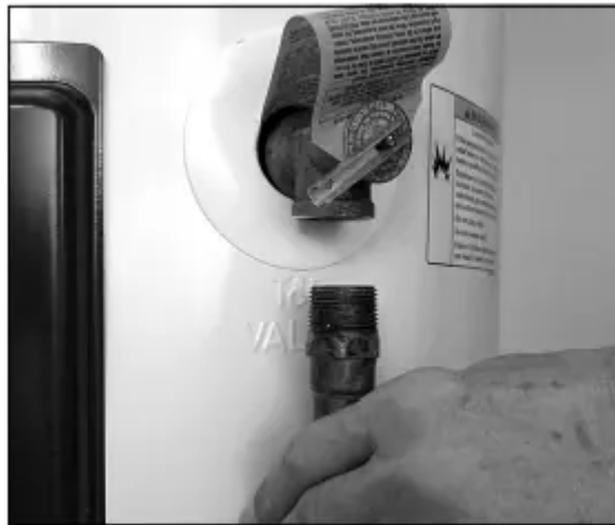
Figure 11 - Removing the T&P Relief Valve discharge pipe.
