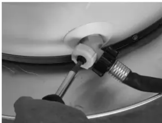
Figure 10 - Draining the old water heater.
