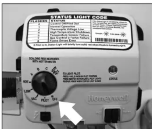
Figure 40 - Turn gas control/temperature knob OFF.
