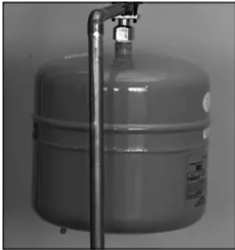
Figure 13 - A Thermal Expansion Tank helps protect the home's plumbing system from pressure spikes.
