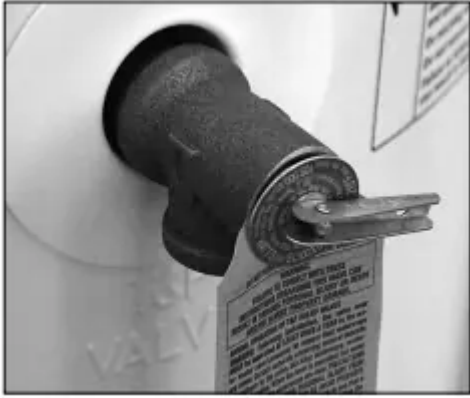
Figure 25 - Temperature and Pressure Relief Valve
