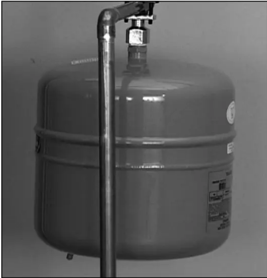
Figure 5 - A Thermal Expansion Tank helps protect the home's plumbing system from pressure spikes
