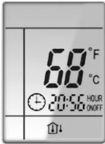
Room Temperature Display
