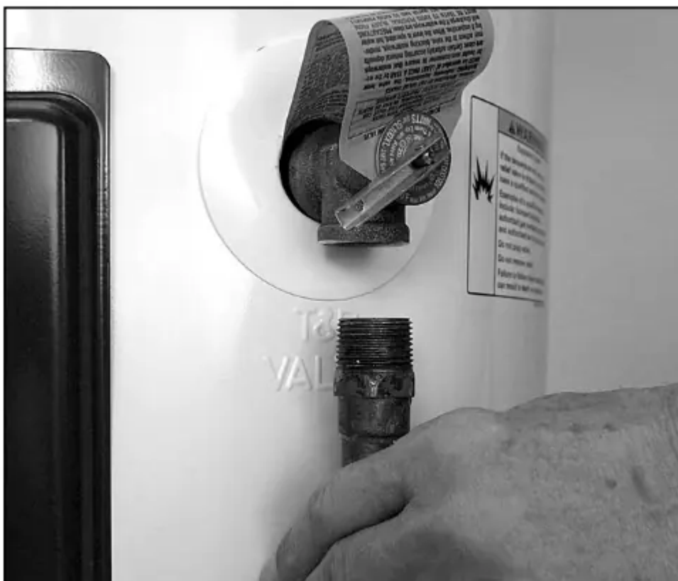
Figure 11 - Removing the T&P Relief Valve discharge pipe.
