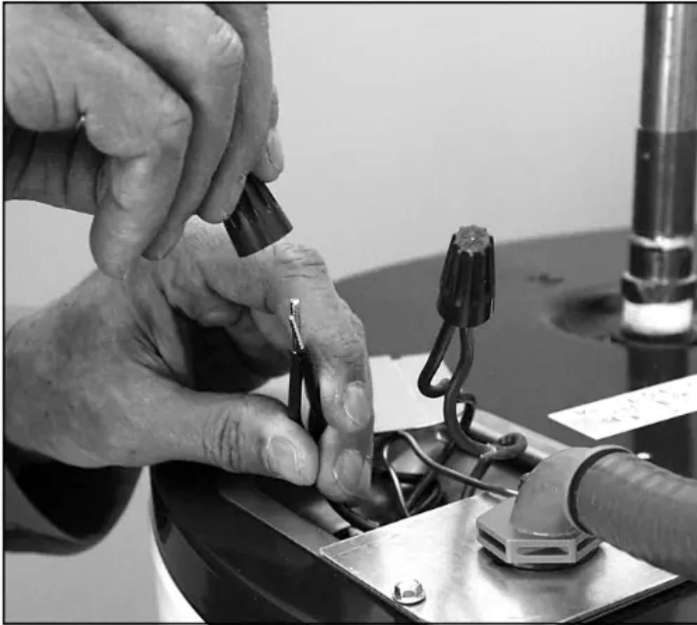
Figure 19 - Connecting the electrical wires.
