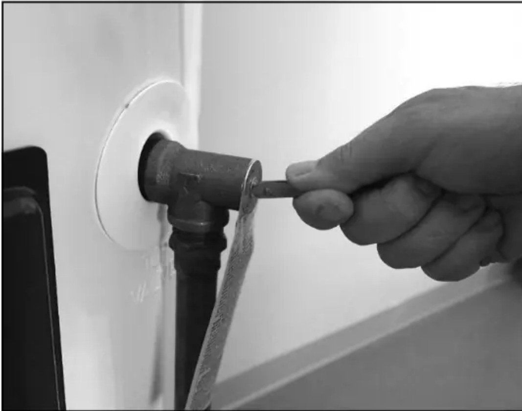
Figure 38 - T&P Relief Valve
