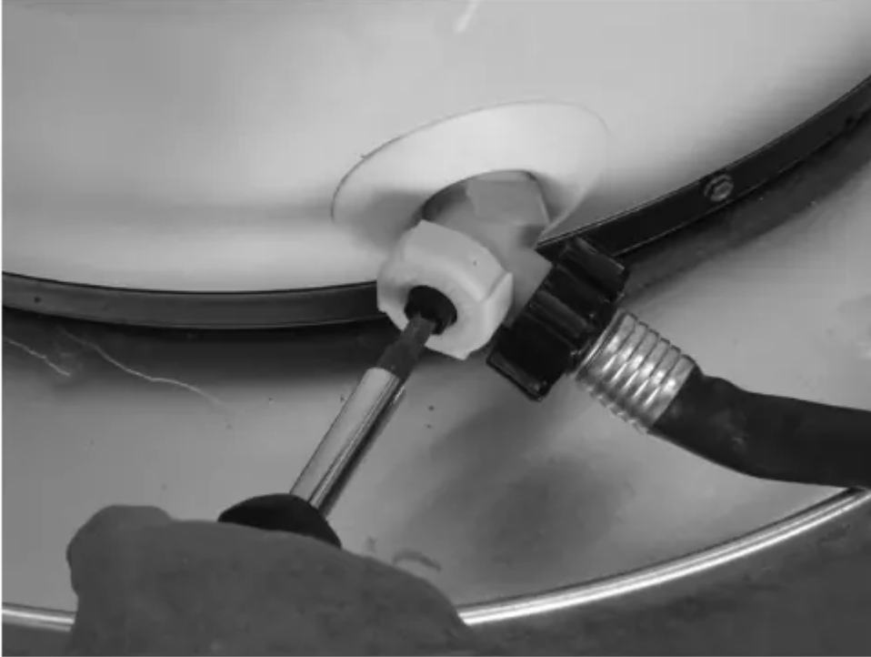
Figure 10 - Draining the old water heater.
