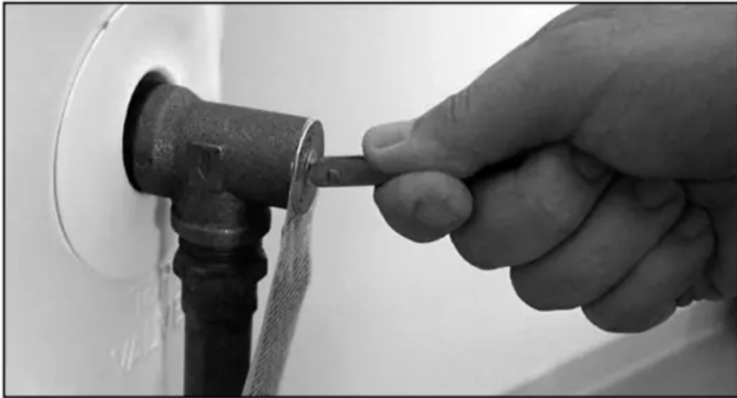
Figure 45 - T&P Relief Valve.
