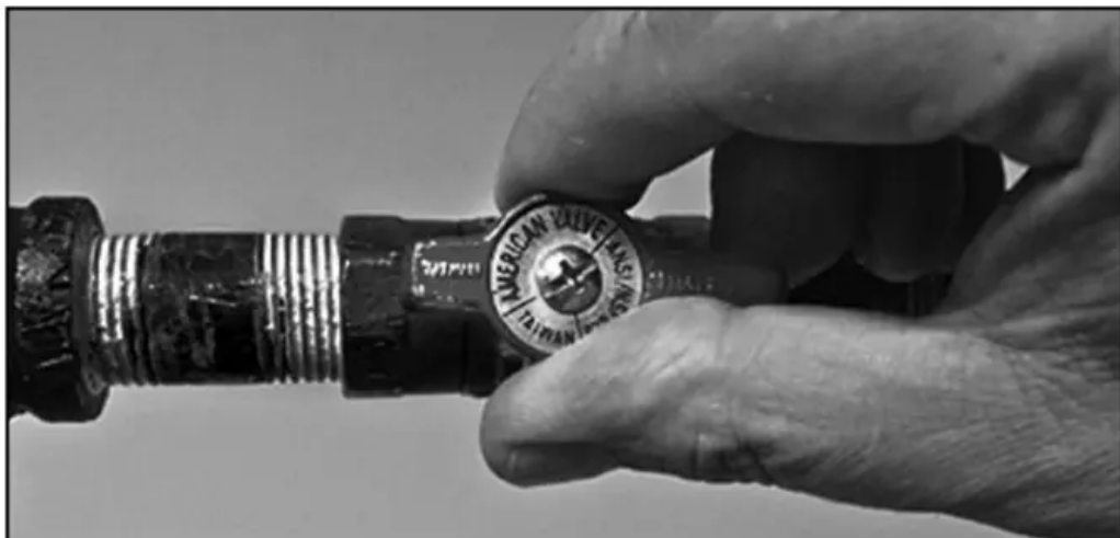
Figure 58 - Gas valve in "on" position.
