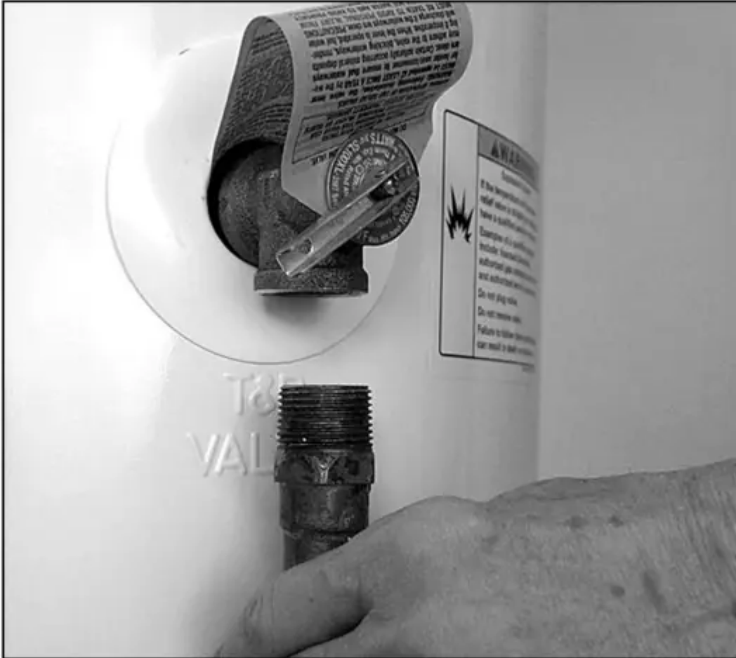
Figure 21 - Removing the T&P Relief Valve discharge pipe.
