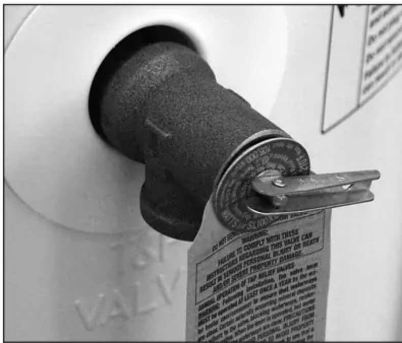
Figure 25 - Temperature and Pressure Relief Valve
