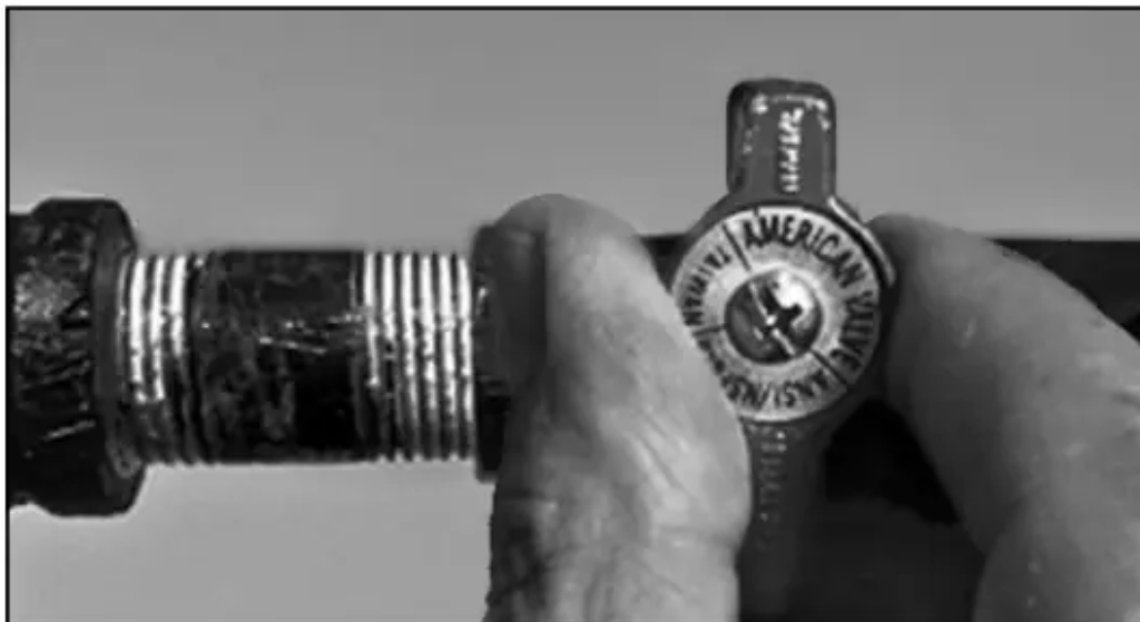
Figure 50 - Gas valve in "off" position.
