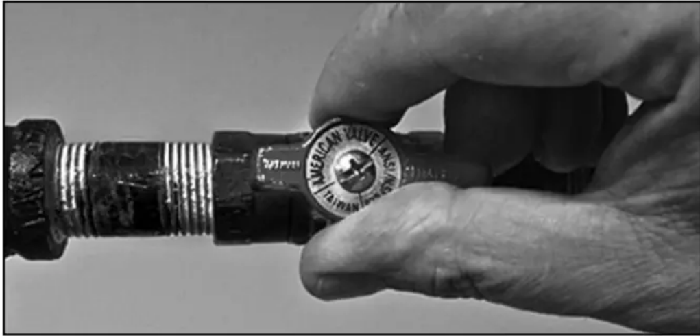
Figure 32 - Gas valve in "on" position
