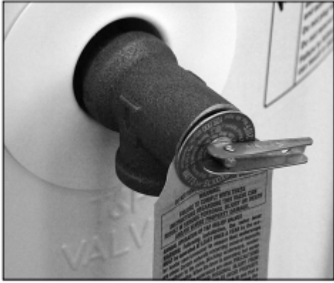
Figure 25 - Temperature and Pressure Relief Valve
