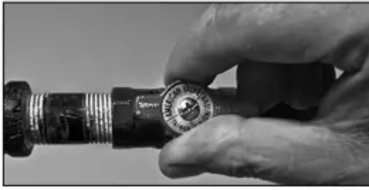
Figure 58 - Gas valve in "on" position.
