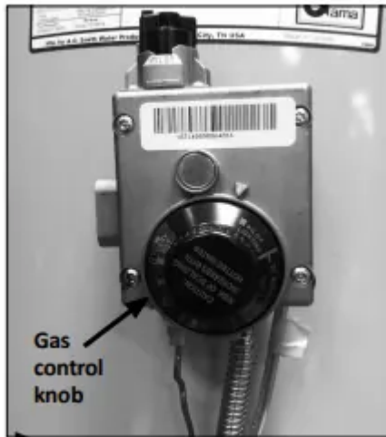
Figure 17 - Turn gas control/temperature knob OFF.
