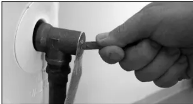
Figure 45 - T&P Relief Valve.
