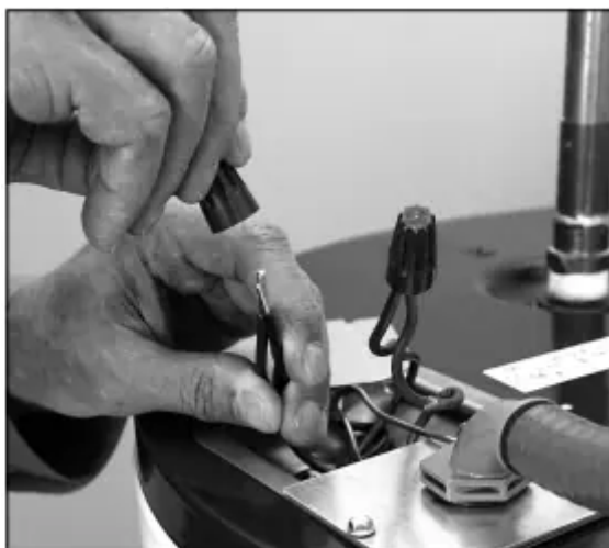
Figure 19 - Connecting the electrical wires
