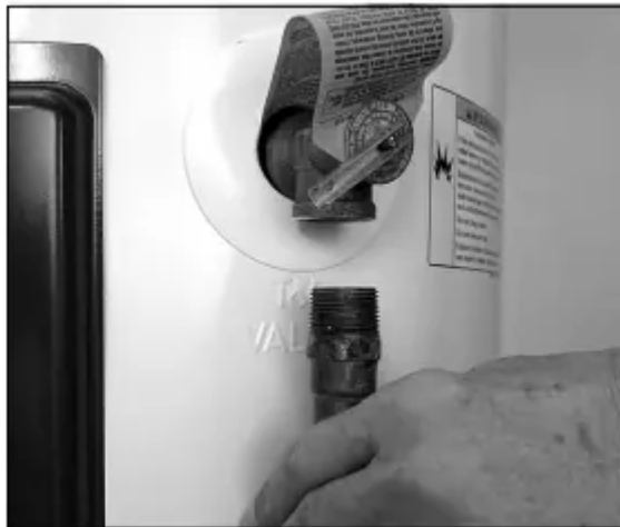
Figure 11 - Removing the T&P Relief Valve discharge pipe.
