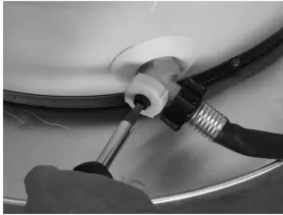
Figure 10 - Draining the old water heater.
