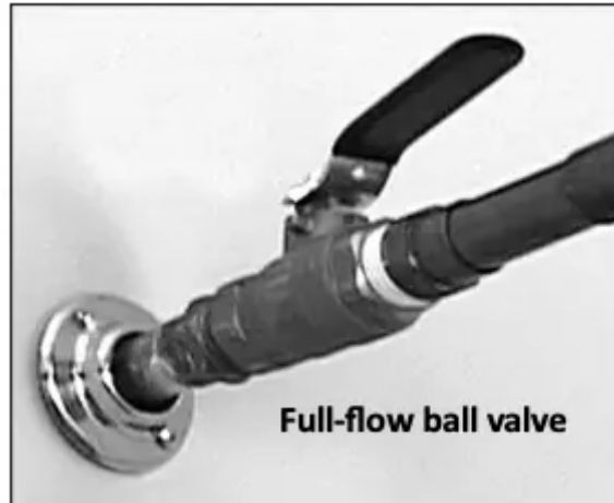
Figure 17 - Fully open the cold water supply valve.
