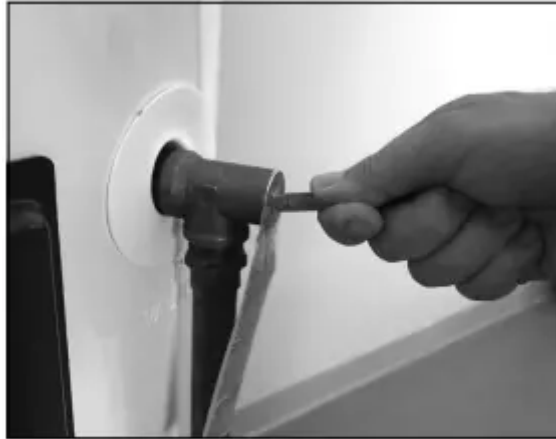
Figure 38 -T&P Relief Valve
