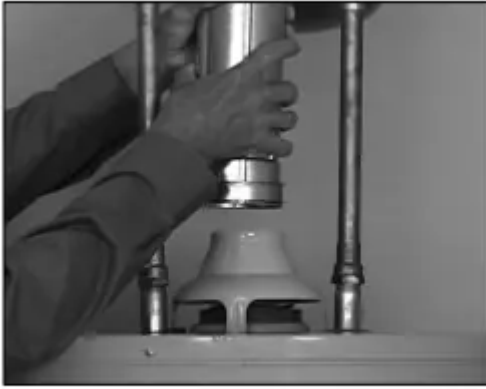
Figure 22 - Disconnect the vent pipe from the draft hood.
