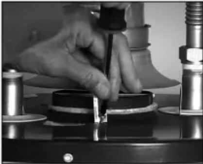
Figure 30 - Install the new draft hood and secure with screws.
