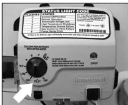
Figure 33 - Gas control/valve.
