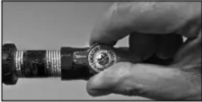
Figure 58 - Gas valve in "on" position.
