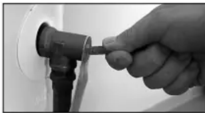
Figure 45 - T&P Relief Valve.
