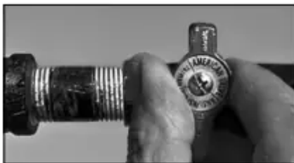
Figure 50 - Gas valve in “off” position.
