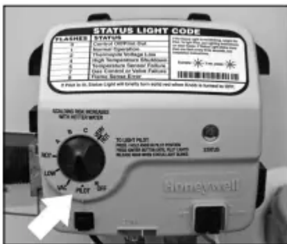
Figure 48 - Gas control/valve.
