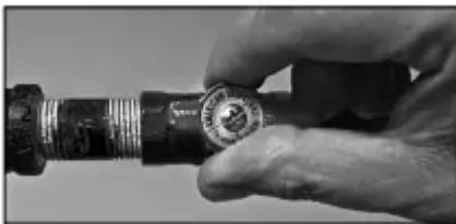
Figure 32 - Gas valve in "on" position
