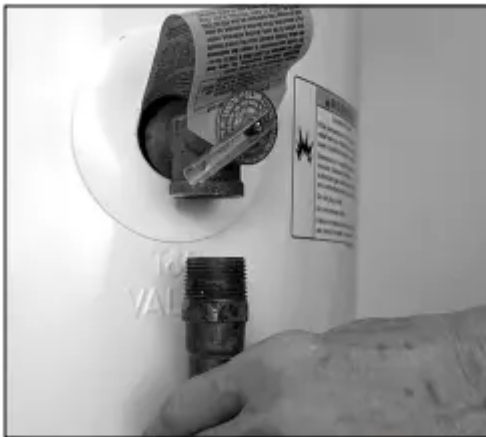
Figure 21 - Removing the T&P Relief Valve discharge pipe.
