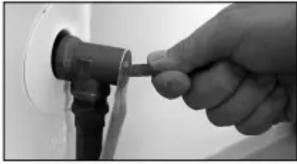
Figure 45 - T&P Relief Valve.
