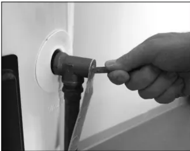
Figure 38 - T&P Relief Valve
