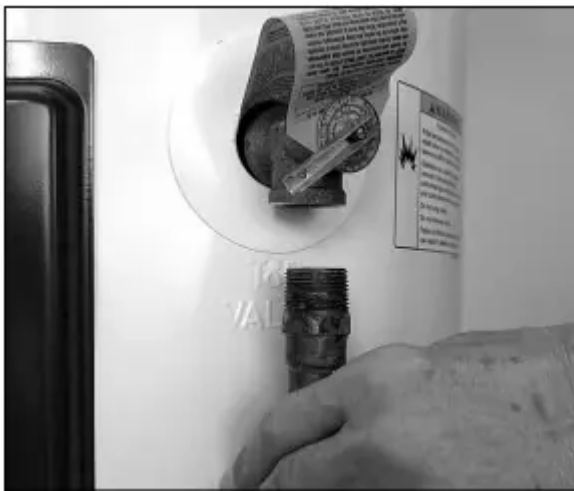
Figure 11 - Removing the T&P Relief Valve discharge pipe.
