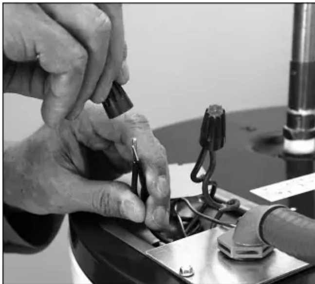
Figure 19 - Connecting the electrical wires.
