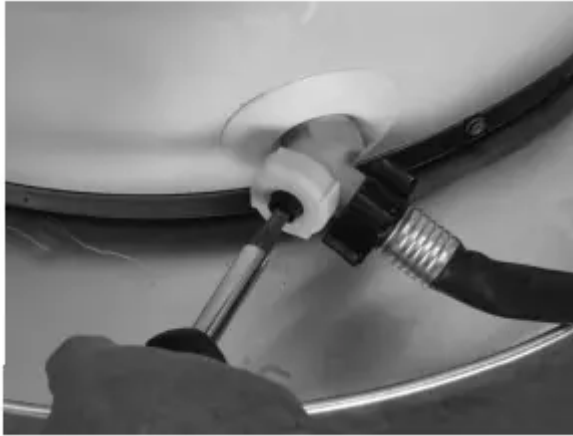
Figure 10 - Draining the old water heater.
