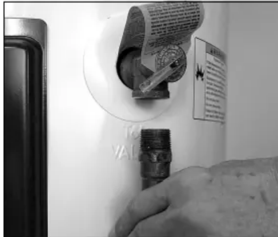
Figure 11 - Removing the T&P Relief Valve discharge pipe.
