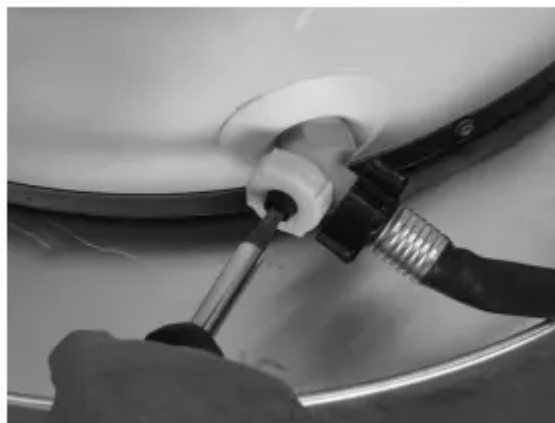
Figure 10 - Draining the old water heater.
