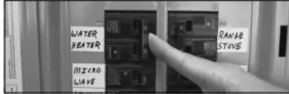
Figure 24 - Circuit Breaker
