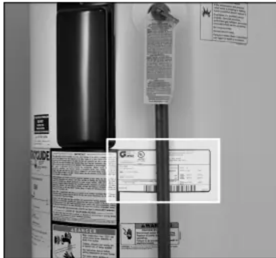
Figure 18 - The water heater's electrical requirements can be determined from the data plate.
