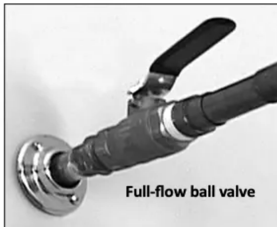
Figure 17 - Fully open the cold water supply valve.
