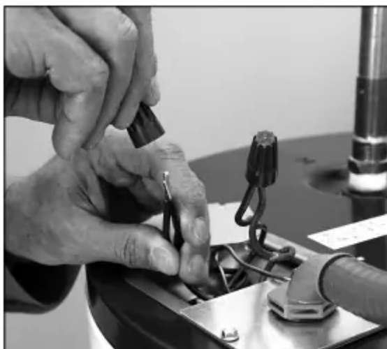
Figure 19 - Connecting the electrical wires.
