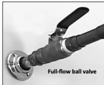
Fully open the cold water supply valve.
