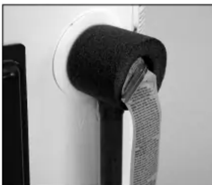
Make sure the insulation does not interfere with the T&P Relief Valve's operation.
