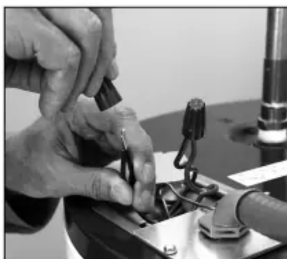
Connecting the electrical wires.
