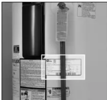
The water heater's electrical requirements can be determined from the data plate.
