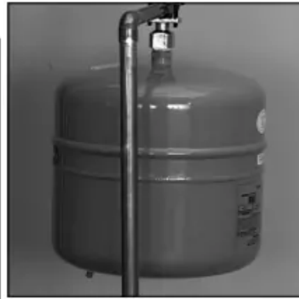
The Thermal Expansion Tank should be pressurized with air, to match the home's incoming water pressure.
