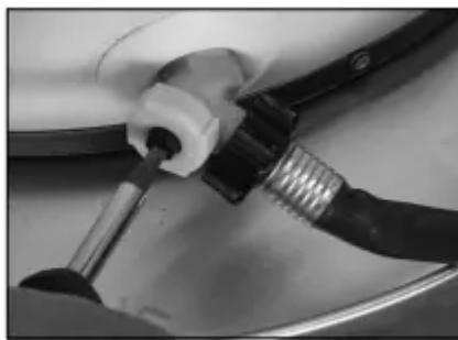
Draining the old water heater.
