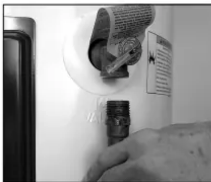
Removing the T&P Relief Valve discharge pipe.
