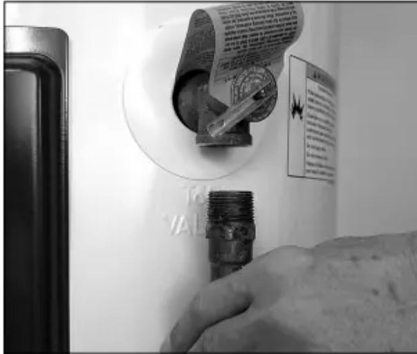
Figure 11 - Removing the T&P Relief Valve discharge pipe .
