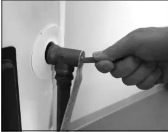
Figure 38 - T&P Relief Valve
