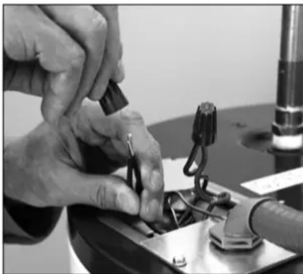
Figure 19 - Connecting the electrical wires.
