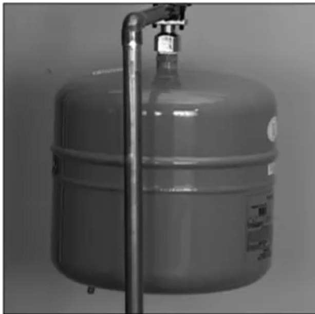
Figure 16 - The Thermal Expansion Tank should be pressurized with air, to match the home's incoming water pressure.
