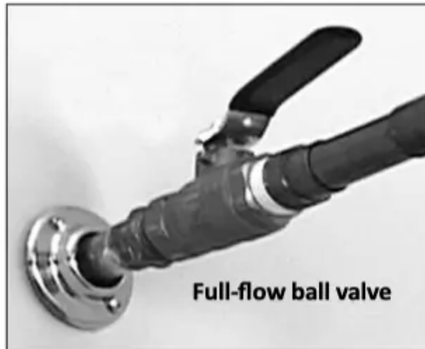
Figure 17 - Fully open the cold water supply valve.
