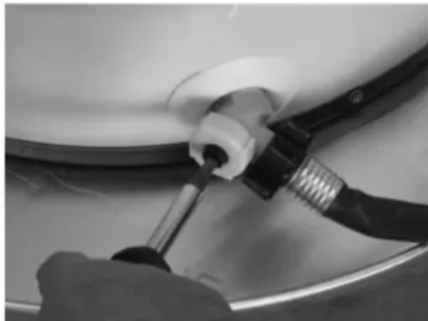
Figure 10 - Draining the old water heater.
