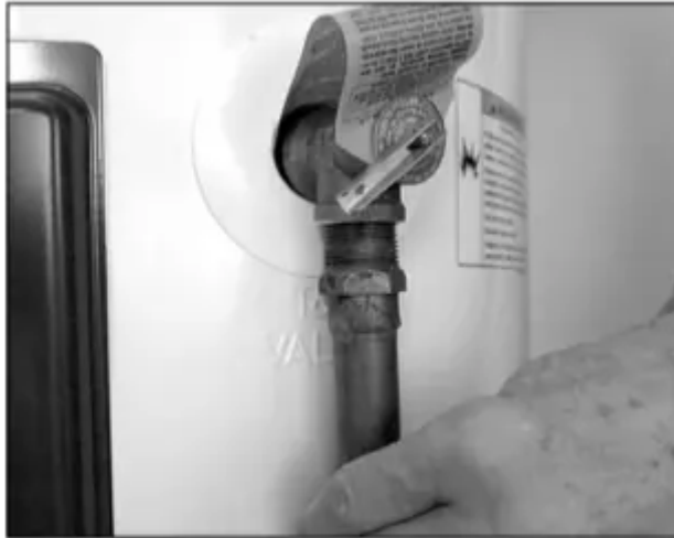
Figure 12 - The T&P Relief Valve discharge pipe must be installed properly and piped to an adequate drain.
