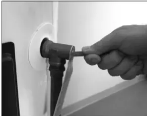
Figure 38 - T&P Relief Valve
