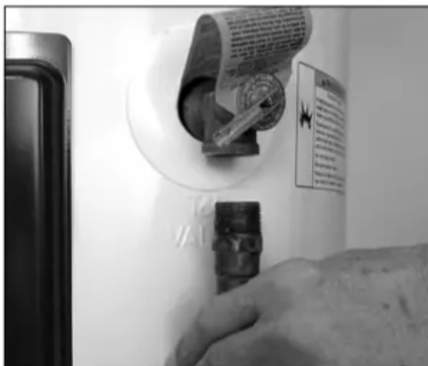
Figure 11 - Removing the T&P Relief Valve discharge pipe.
