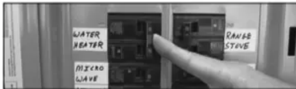
Figure 31 - Circuit Breaker
