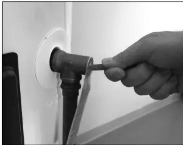
Figure 38 - T&P Relief Valve
