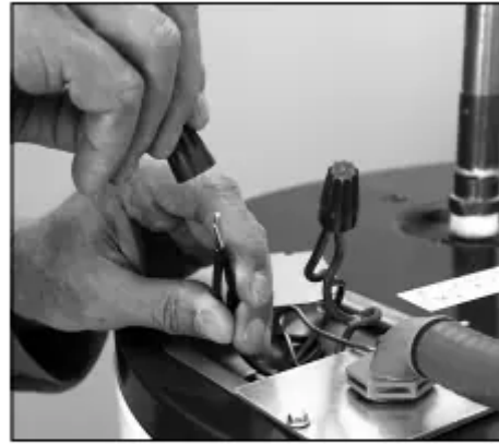
Figure 19 - Connecting the electrical wires.
