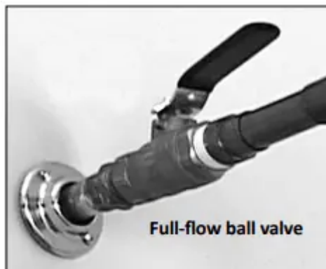
Figure 17 - Fully open the cold water supply valve.
