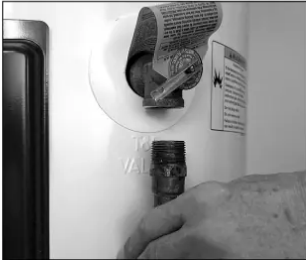
Figure 11 - Removing the T&P Relief Valve discharge pipe.
