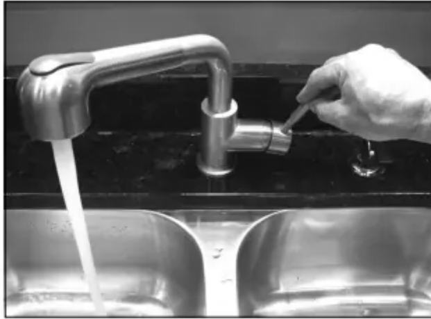
minutes or longer). Figure 9 - Let the hot water run until it is cool.
