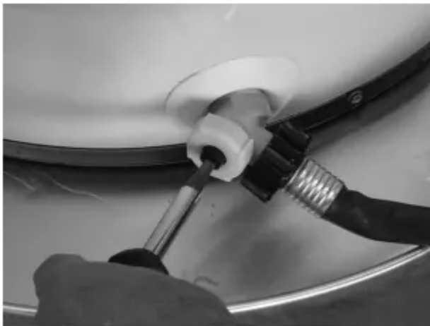
Figure 10 - Draining the old water heater.
