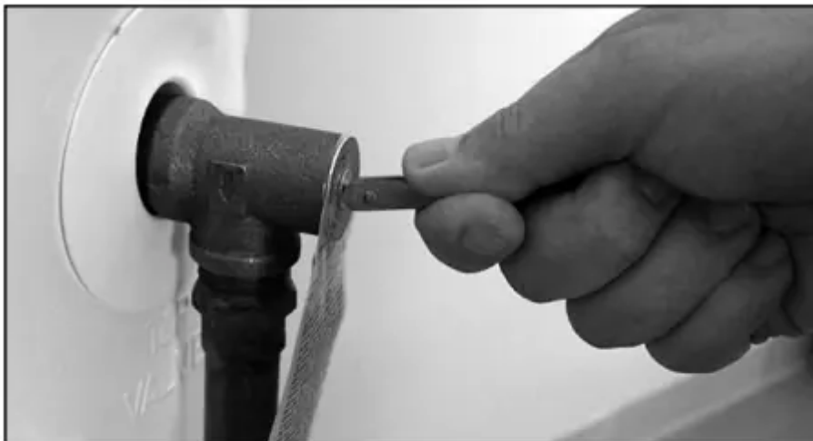
Figure 45 - T&P Relief Valve.
