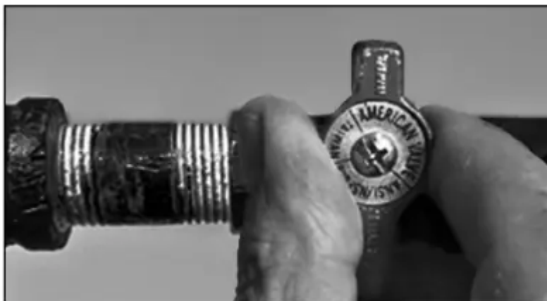
Figure 50 - Gas valve in "off" position.
