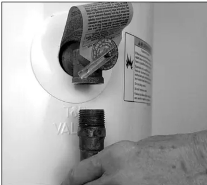
Figure 21 - Removing the T&P Relief Valve discharge pipe.
