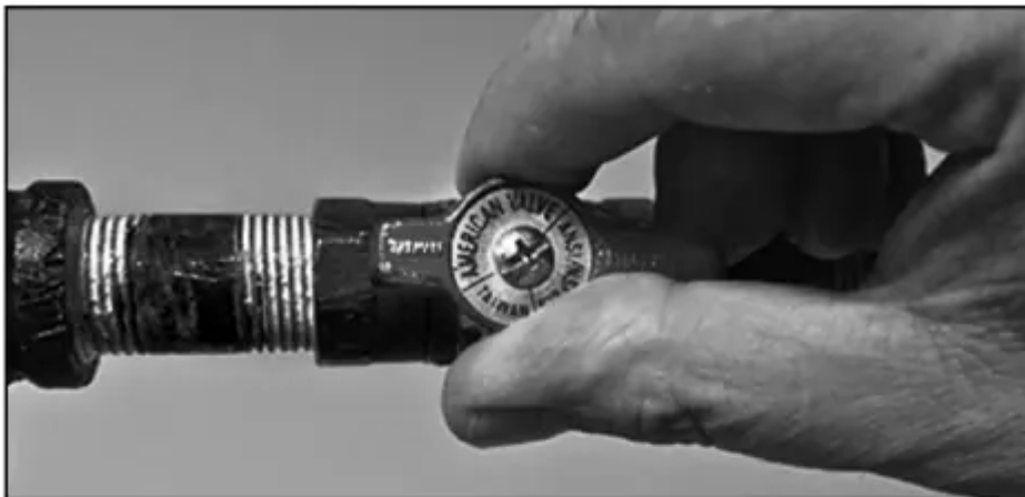
Figure 32 - Gas valve in "on" position
