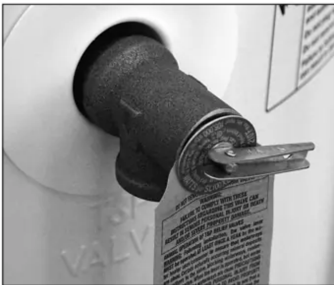
Figure 25 - Temperature and Pressure Relief Valve
