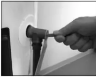
Figure 38 - T&P Relief Valve
