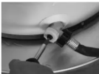
Figure 10 - Draining the old water heater.
