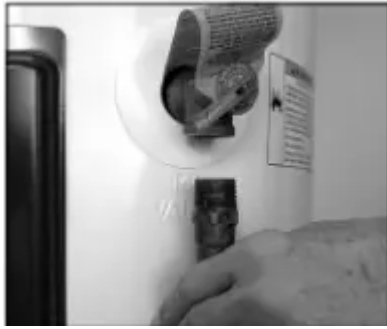
Figure 11 - Removing the T&P Relief Valve discharge pipe.
