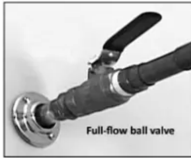
Figure 17 - Fully open the cold water supply valve.
