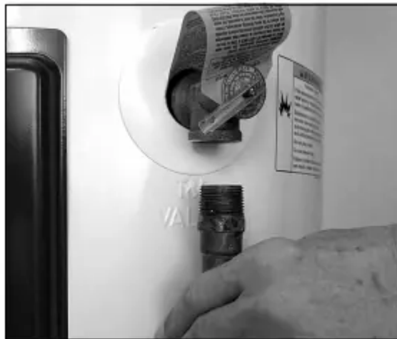
Figure 11 - Removing the T&P Relief Valve discharge pipe.
