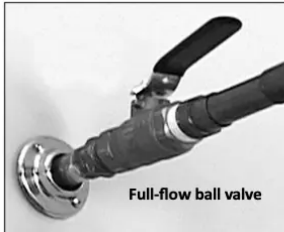
Figure 17 - Fully open the cold water supply valve.
