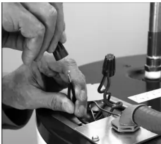
Figure 19 - Connecting the electrical wires.
