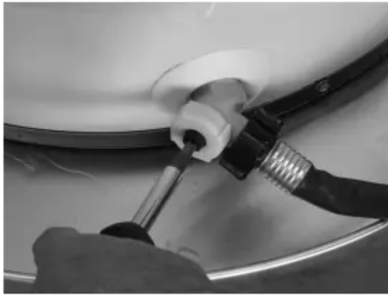
Figure 10 - Draining the old water heater.
