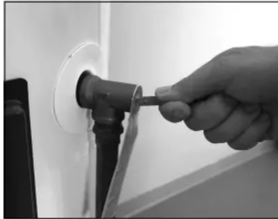
Figure 38 - T&P Relief Valve
