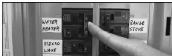
Figure 24 - Circuit Breaker
