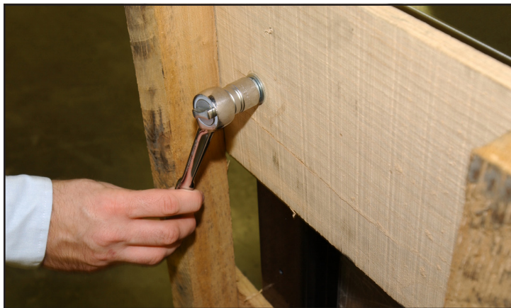
Removing skid from bottom of cabinet.
