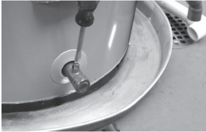
Figure 10 - Draining the old water heater.
