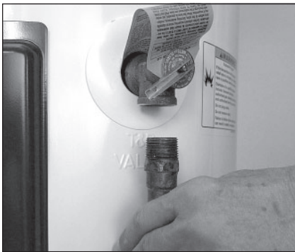
Figure 11 - Removing the T&P Relief Valve discharge pipe.
