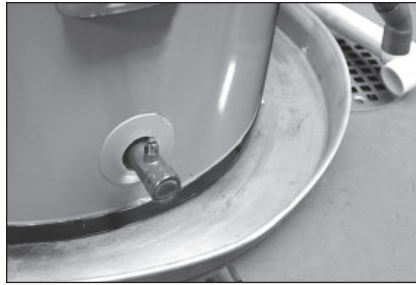
Figure 6 - A suitable drain pan piped to an adequate drain can help protect flooring from leaks and drips.
