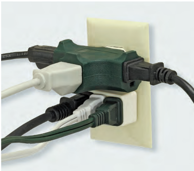
Be careful not to overload a circuit
