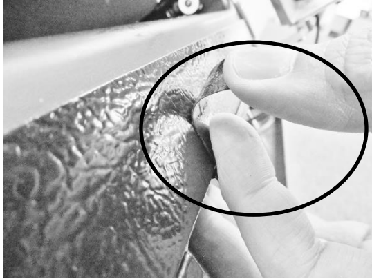
Peel away from cabinet flange
