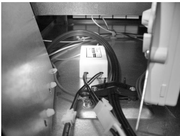
Place the power supply between the main power board and condenser fan as far forward as possible.
