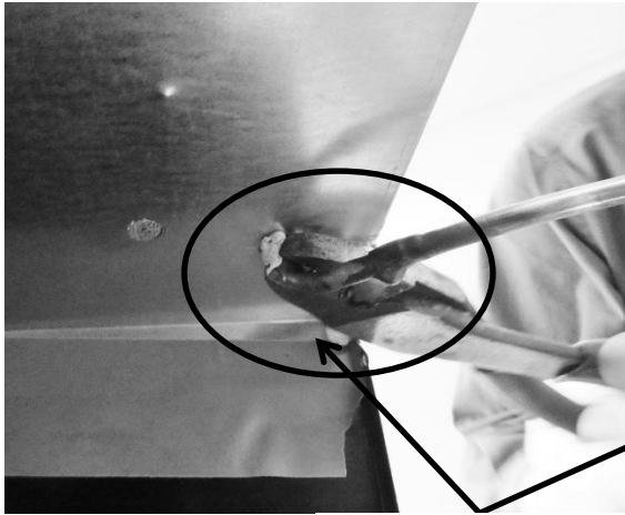
Cut away suction line at the above locations.
