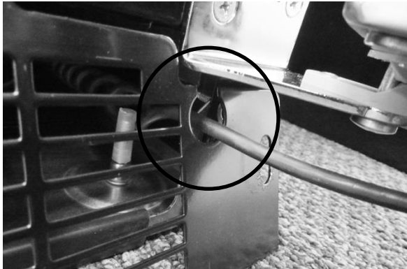
CORRECT wire position- Inside grommet.
