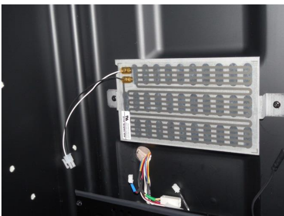
A replacement heater will appear as seen to the left. The heater will come attached to a replacement bracket.
