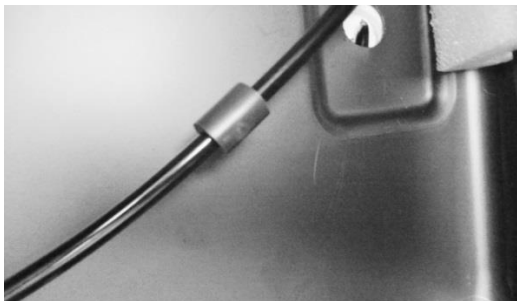
Install vibration isolator on heat exchanger assembly behind evaporator.
