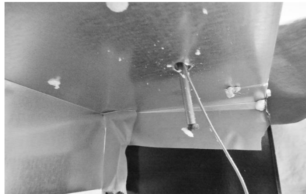
Extend new assembly through the hole. Make sure ends are capped.
