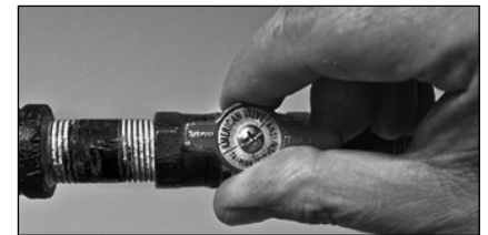
Figure 42 - Gas valve in "on" position.
