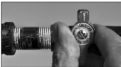
Figure 40 - Gas valve in "off" position
