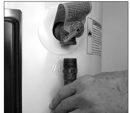
Figure 12 - Removing the T&P Relief Valve discharge pipe.
