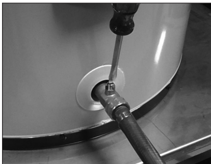
Figure 11 - Draining the old water heater.
