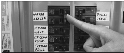
Figure 42 - Circuit Breaker.
