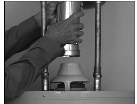
Figure 22 - Disconnect the vent pipe from the draft hood.
