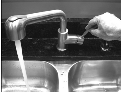
Figure 41 - Let the hot water run until it is cool.
