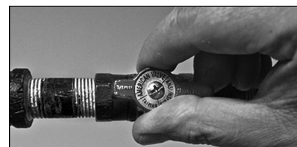
Figure 58 - Gas valve in “on” position.
