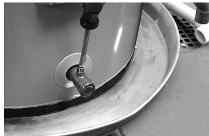
Figure 20 - Draining the old water heater.
