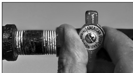
Figure 50 - Gas valve in “off” position.
