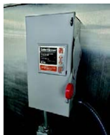
Single Unit Independently Fused Power Supply Line
