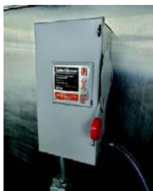
Combi-Duo Unit Independently Fused Power Supply Line
