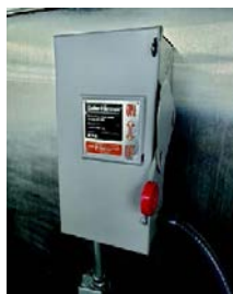
Combi-Duo Unit Independently Fused Power Supply Line
