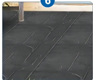
Spray sealing protective agent
