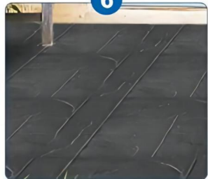
Spray sealing protective agent
