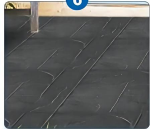
Spray sealing protective agent
