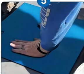
Stamp the concrete
