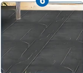
Spray sealing protective agent
