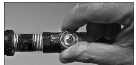
Figure 50 - Gas valve in “on” position.
