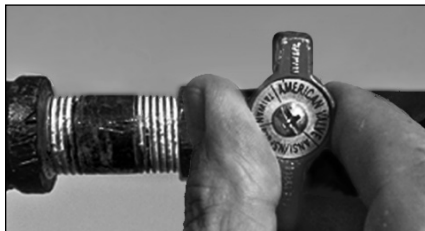
Figure 46 - Gas valve in “off” position.
