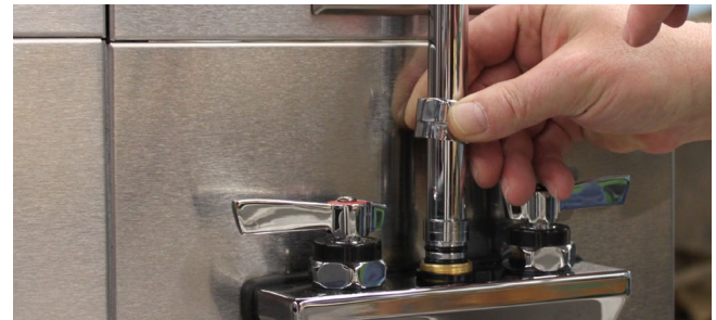
14. Insert the bottom of the spout (goose neck spout shown) into center opening of faucet body.
