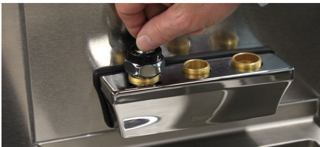
11. Insert hot water valve assembly in the left opening in the faucet body. Note: Hot and cold valves are identified with "Hot" or "Cold" stamped in valve body. Turn chrome nut on top of valve to tighten. Note: Torque spec is 25 ft. lbs.
