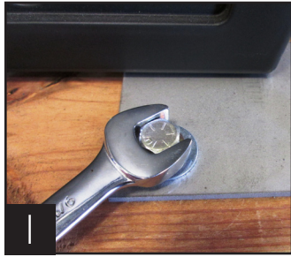
1 Removing bracket from skid.
