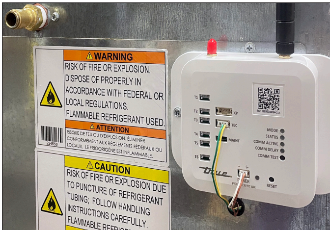
Fig. 2. Wire harness connected to modem. Green/Yellow to TEC; Brown/White to POWER.
