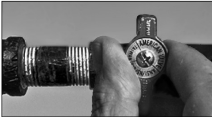
Figure 50 - Gas valve in "off" position.
