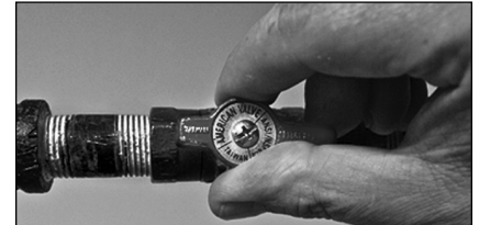
Figure 58 - Gas valve in "on" position.
