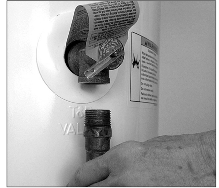
Figure 21 - Removing the T&P Relief Valve discharge pipe.
