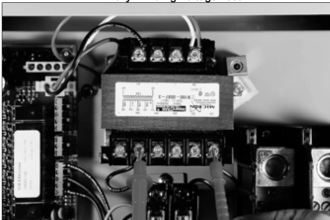
Figure 33. 120 VAC Control Circuit Winding Voltage Tests
