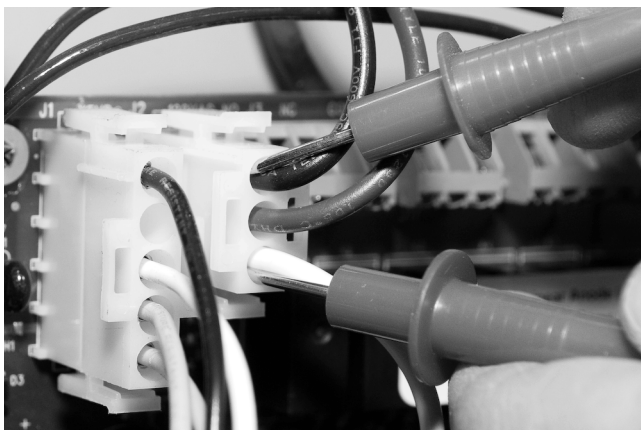
Figure 47. Checking for 120 VAC Power
