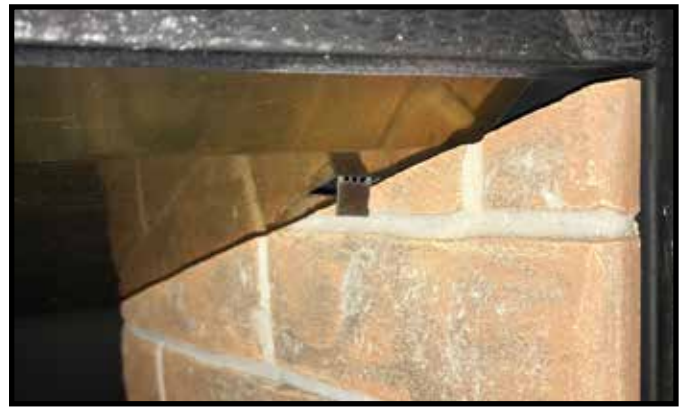
Figure 7 Right Refractory Handbend Tab
