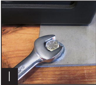
1 Removing bracket from skid.
