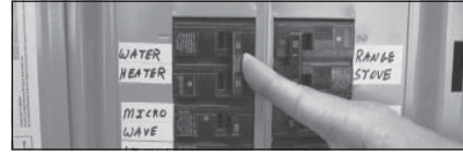
Figure 22 - Circuit Breaker
