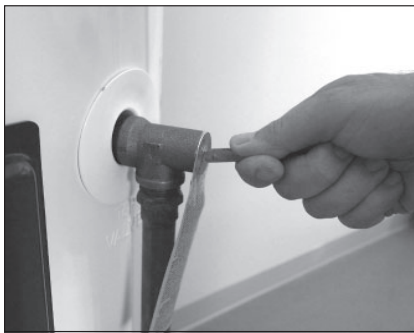
Figure 40 - T&P Relief Valve
