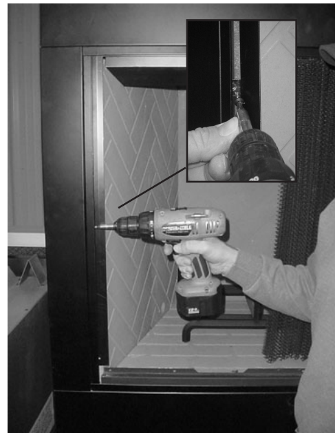
Figure 5 - Fastening the Side Filler
