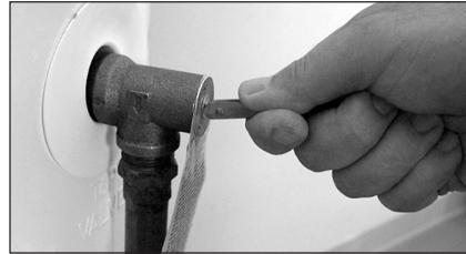
Figure 42 - T&P Relief Valve.
