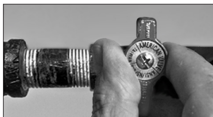
Figure 45 - Gas valve in "off" position.
