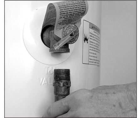
Figure 21 - Removing the T&P Relief Valve discharge pipe.
