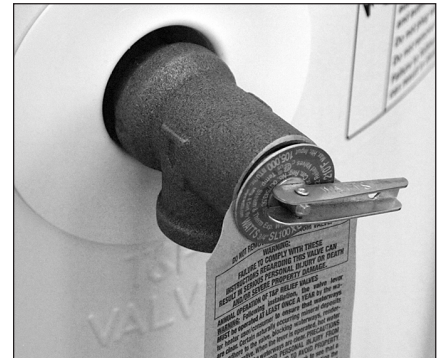
Figure 24 - Temperature and Pressure Relief Valve
