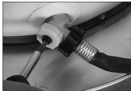
Figure 20 - Draining the old water heater.
