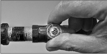
Figure 49 - Gas valve in “on” position.
