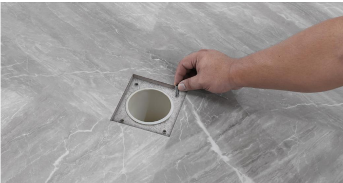
4. Put the screws into the holes.
