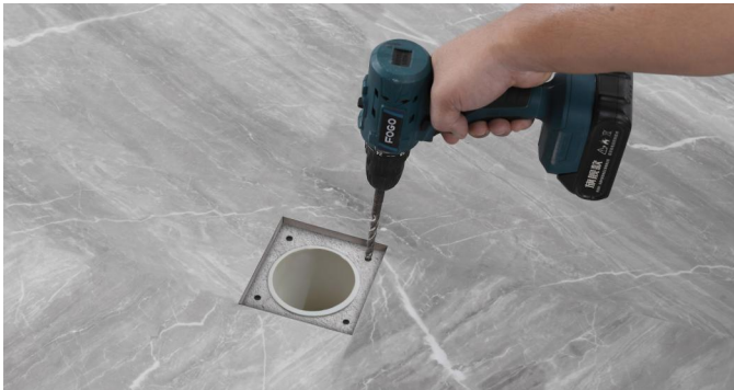
3. Take off the fixed disk and drill four holes for screws.
