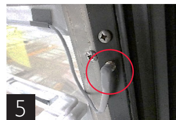
Light cord installed
