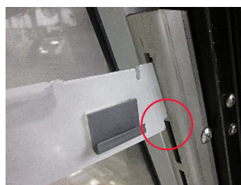
Top notch installed (gap)
