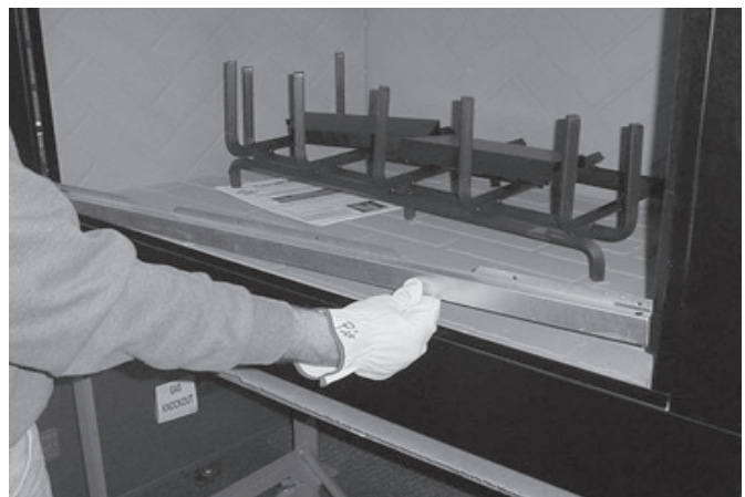
Figure 1 - Install the Door Track
