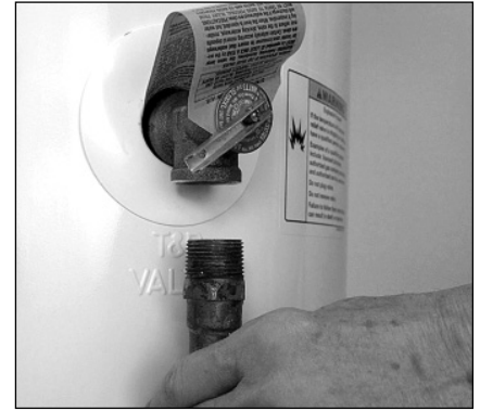
Figure 21 - Removing the T&P Relief Valve discharge pipe.
