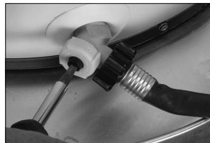
Figure 12: Draining the old water heater.
