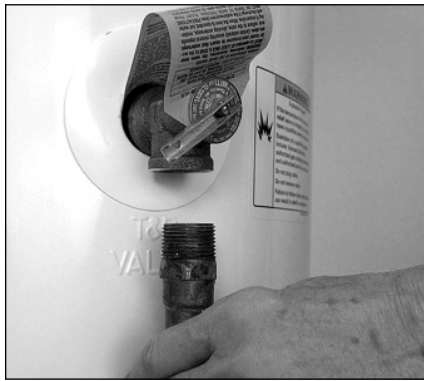
Figure 13: Removing the T&P Relief Valve discharge pipe.
