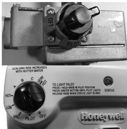
Figure 9: Turn gas control/temperature knob OFF.
