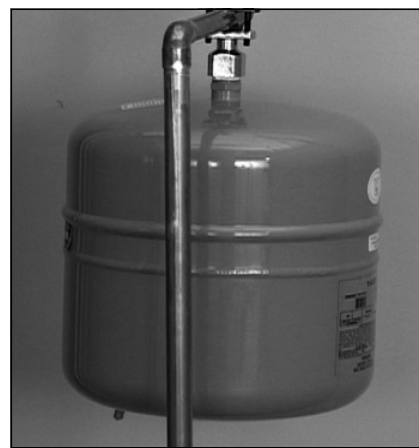
Figure 6: A Thermal Expansion Tank helps protect the home's plumbing system from pressure spikes.
