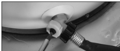
Figure 47: Draining the water heater.
