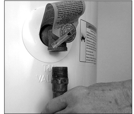
Figure 21 - Removing the T&P Relief Valve discharge pipe.
