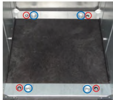
Red = Stabilizing Bolts; Blue = Screw Anchor
