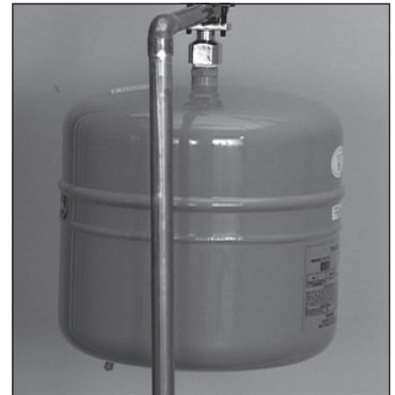
Figure 5 - A Thermal Expansion Tank helps protect the home's plumbing system from pressure spikes.
