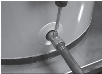
Figure 10 - Draining the old water heater.
