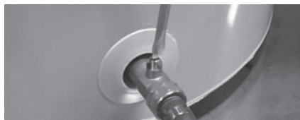
Figure 29 - Drain Valve
