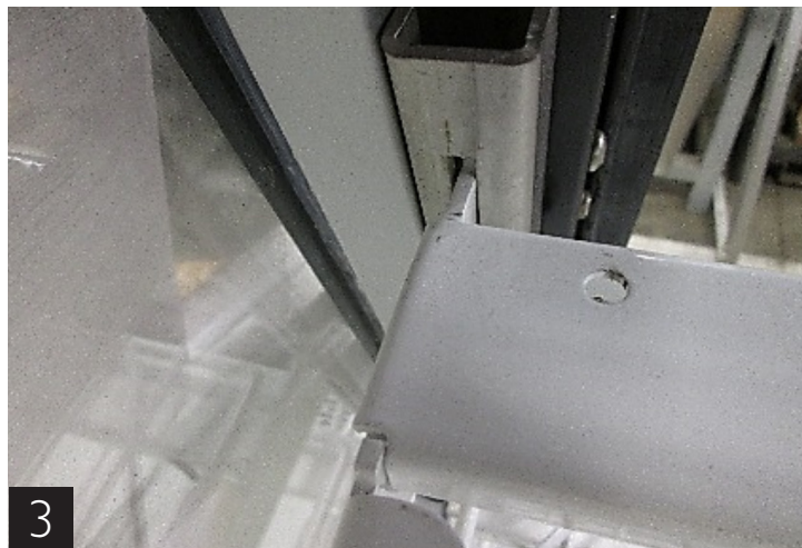
Light assembly installed on shelf support
